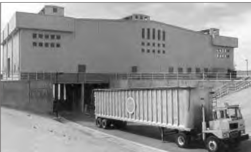
Many transfer stations are multi-level facilities that allow vehicle access at several levels.
