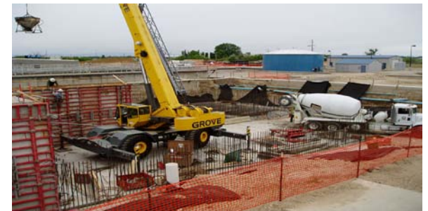
Wastewater construction project.
