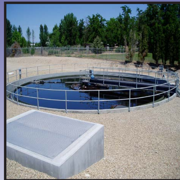
Wastewater treatment facility, Moore, Idaho.
