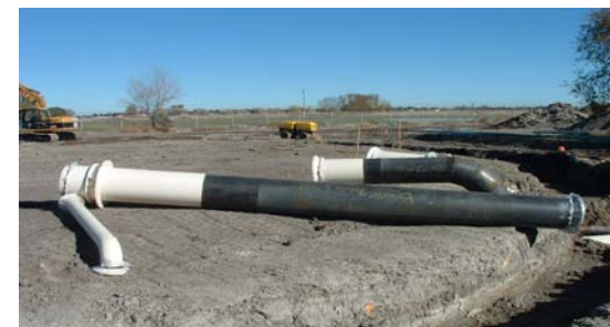
Drinking water construction project.
