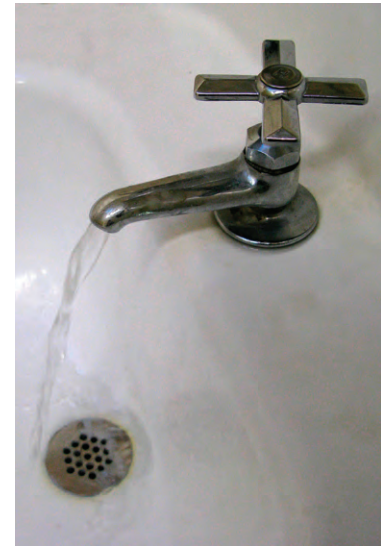
A smooth-nose tap prevents possible contamination of a water sample.
